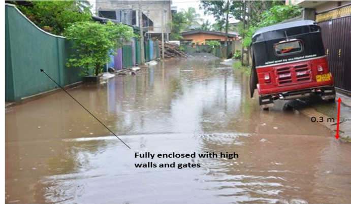
Figure 5: Flood protection measures -entrance elevated barriers and fully covered walls (Date of the image:(September 2022)
